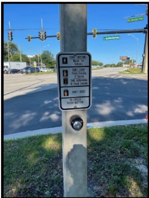
Image 16- Push buttons to the north of S.R. 436 are missing appropriate labels.
