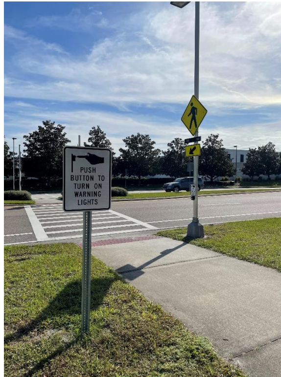
Larger Ped Button signs at International Parkway and Westin Hotel RRFB
